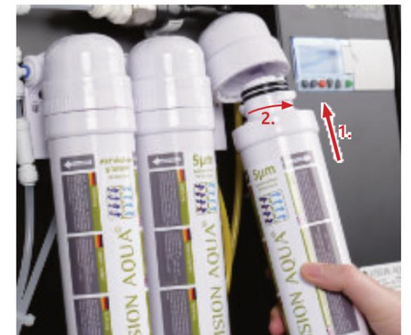
Insert the new filter cartridge into the filter heads by rotating the filter cartridges 90° clockwise. Proceed in the same way for the second PP pre-filter unit.
