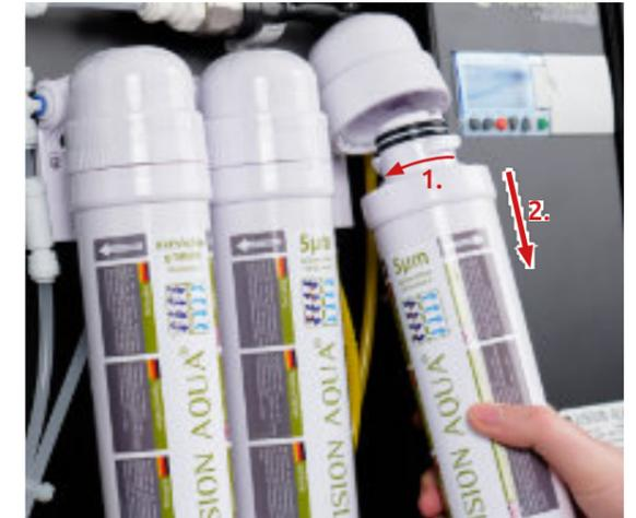
Turn filter cartridge counterclockwise 90° out of the filter head to change the filter unit.
