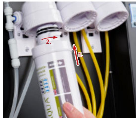
Insert the new filter cartridge into the filter head by rotating the filter cartridge 90° clockwise.
