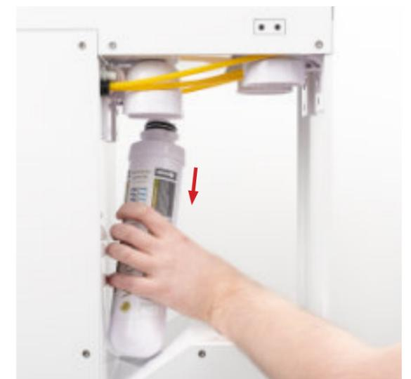
Now you can remove the filter cartridge from the filter head. Install the new post-filters in reverse order.
